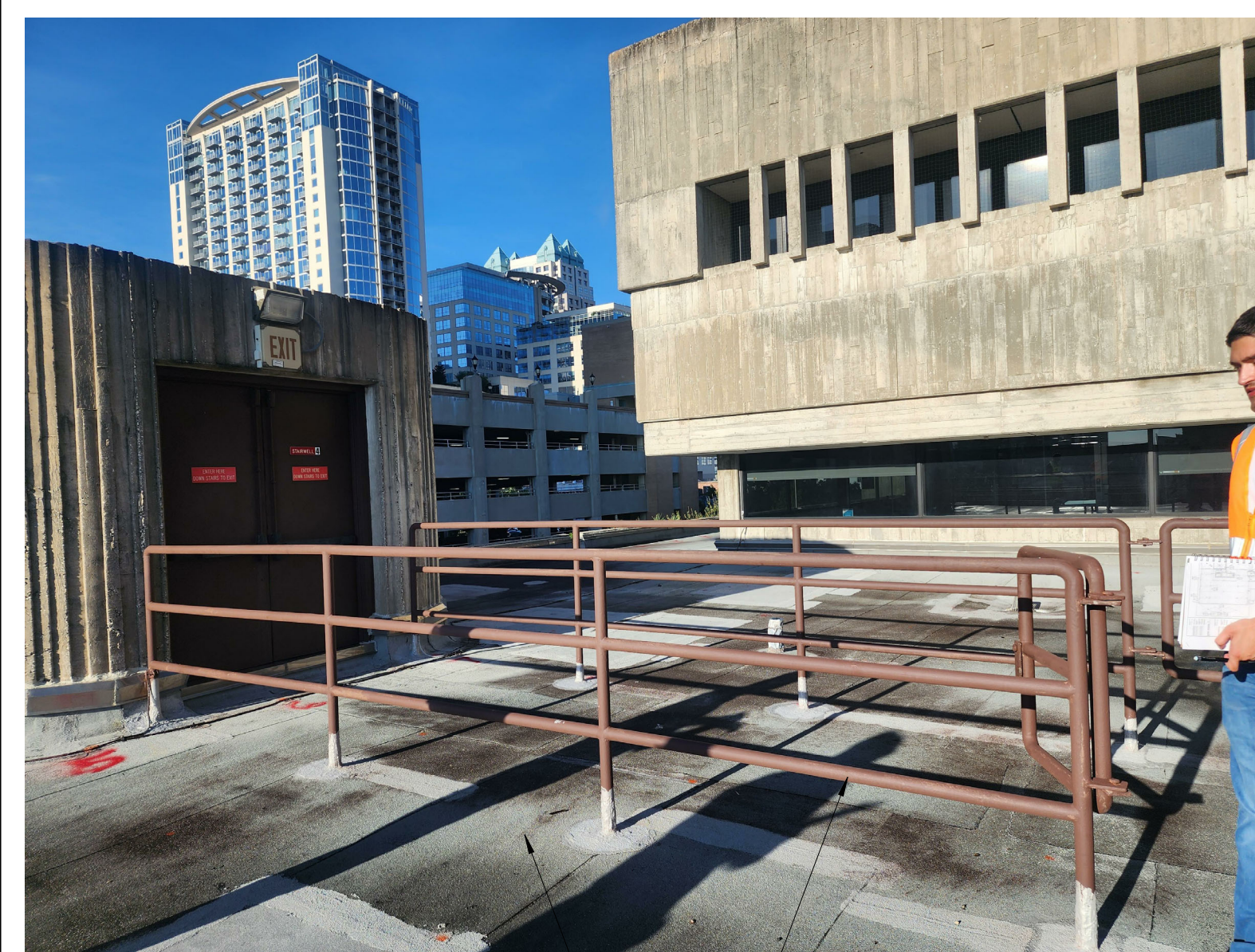
ROOF ACCESS WALKWAY 01
