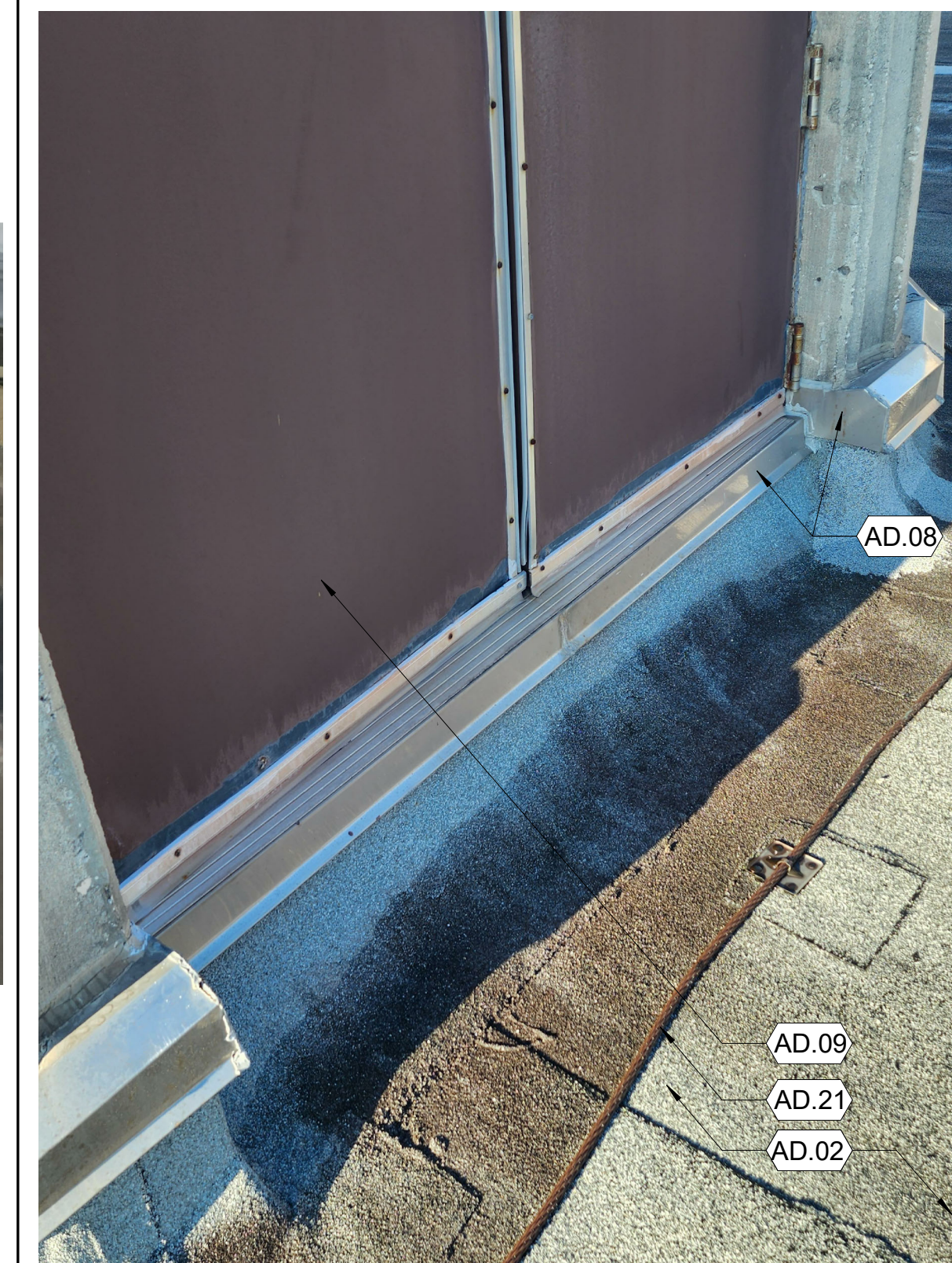
FLASHING AT MECHANICAL DOOR 02
