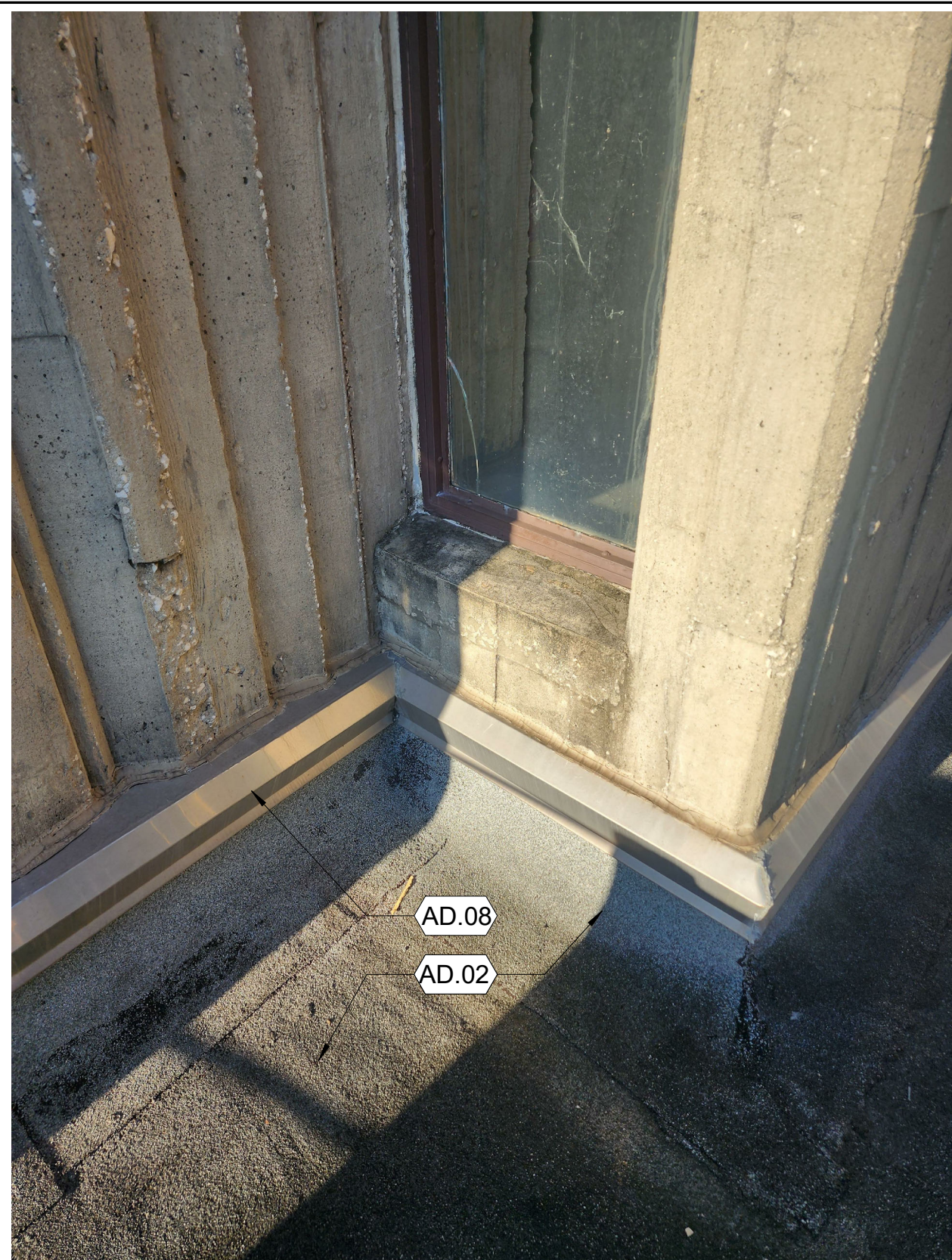
WINDOW SILL AND FLASHING 07
