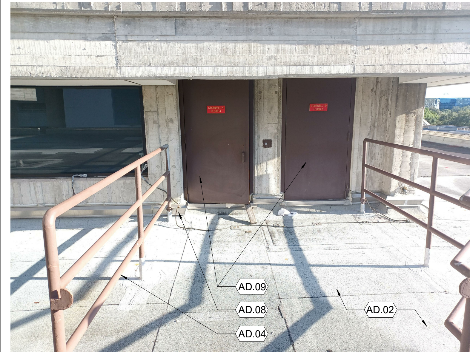
MAIN BUILDING EXIT WITH ACCESS WALKWAY 03
