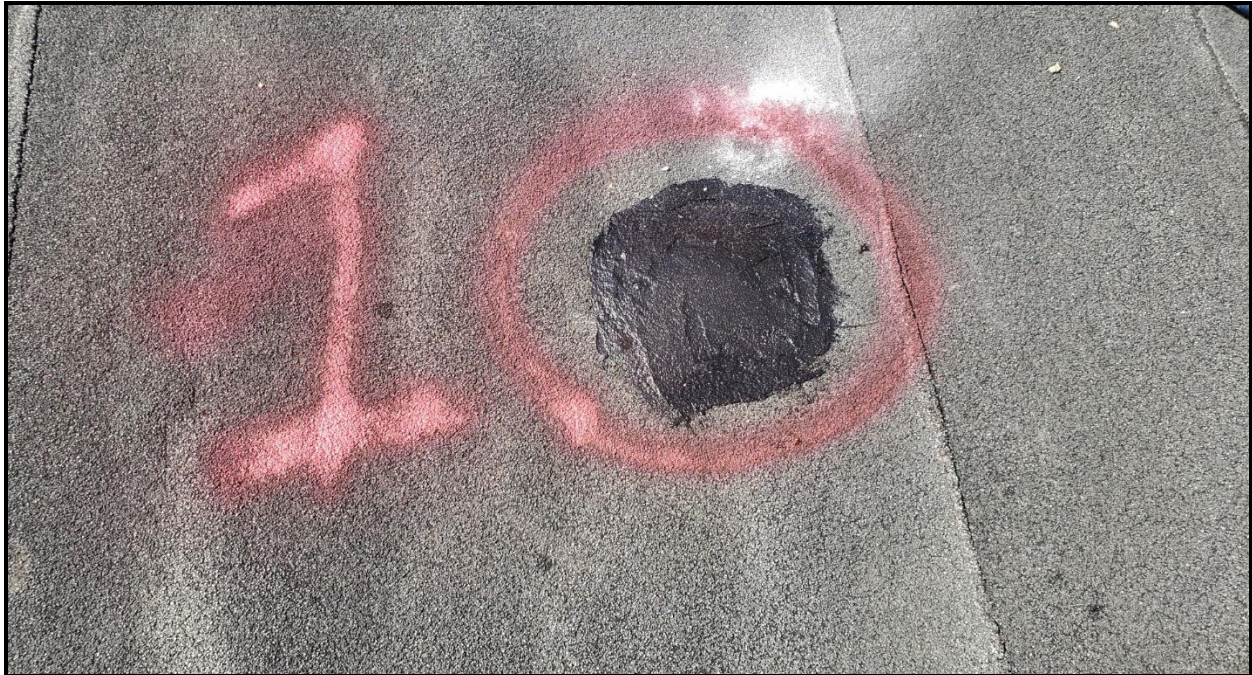
Photo 5: Typical roof core/sample 1 patched
