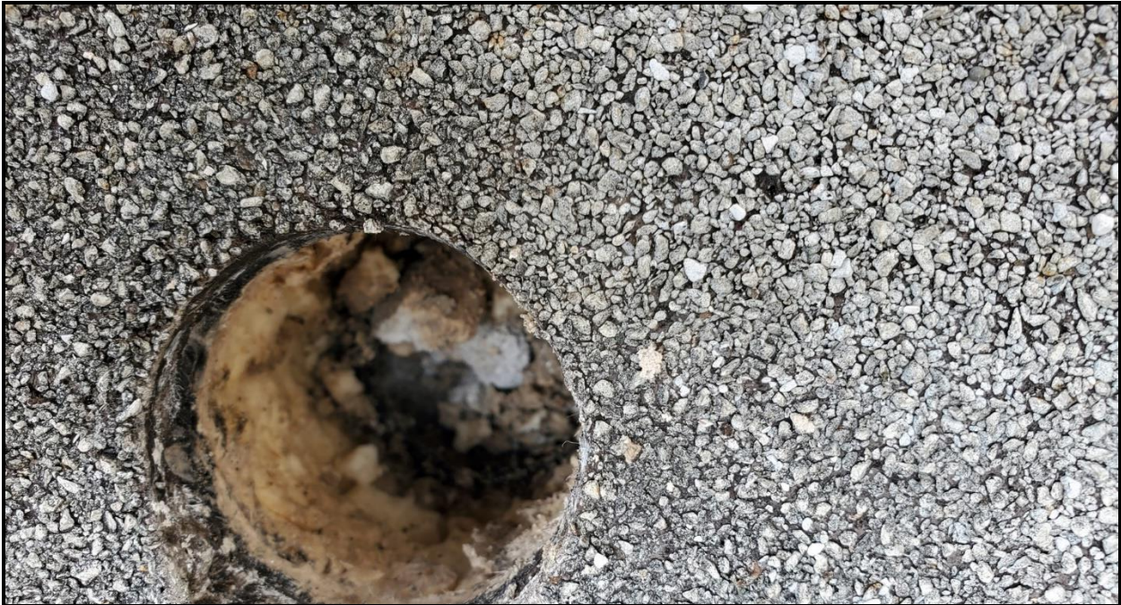
Photo 17: Roof core sample 7
