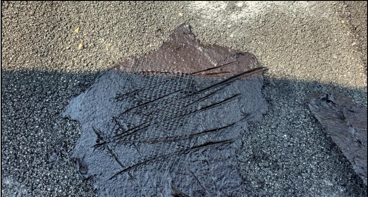
Photo 4: Typical roof patch consisting of 3-ply roof asphalt, 2-ply mesh.
