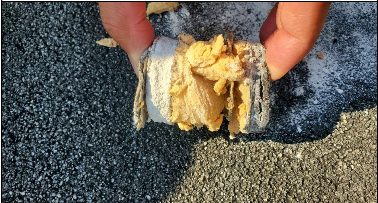
Photo 2: Roof core 1 collected from area 1
