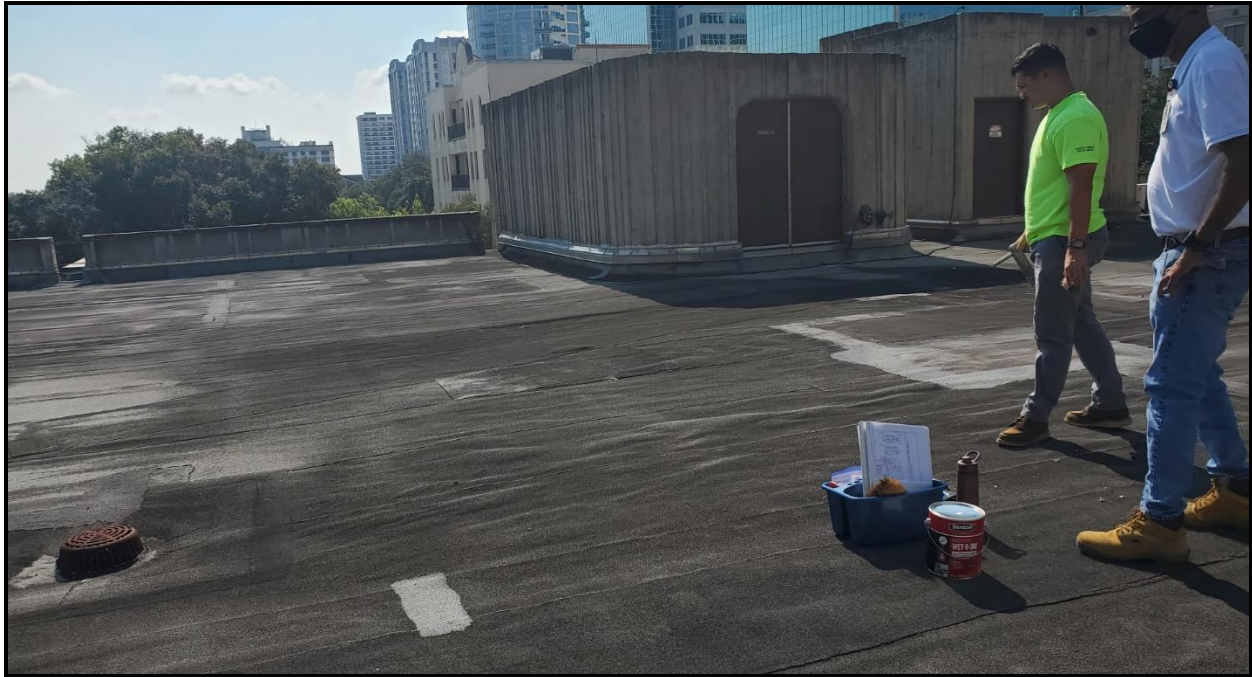
Photo 1: Overall view of roof area 1
