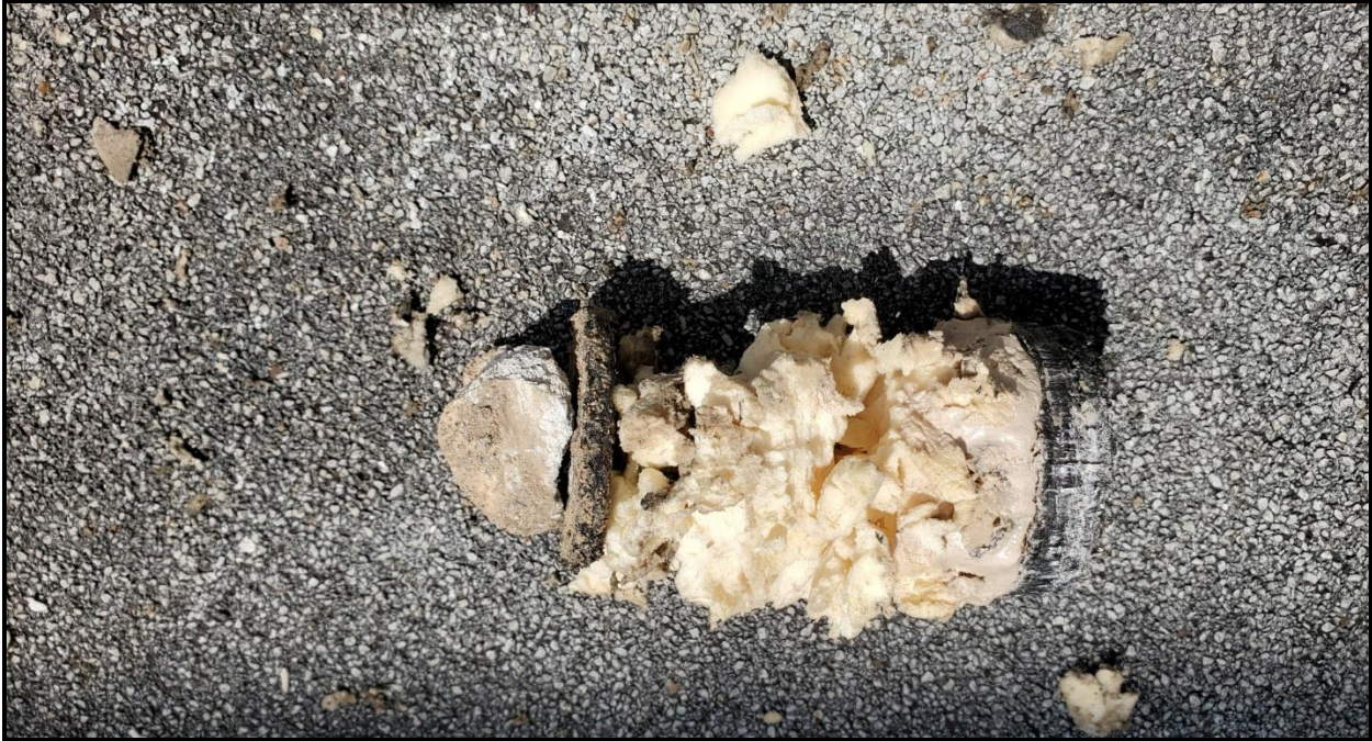
Photo 15: Sample 7 collected from area 3 outside mechanical penthouse entrance
