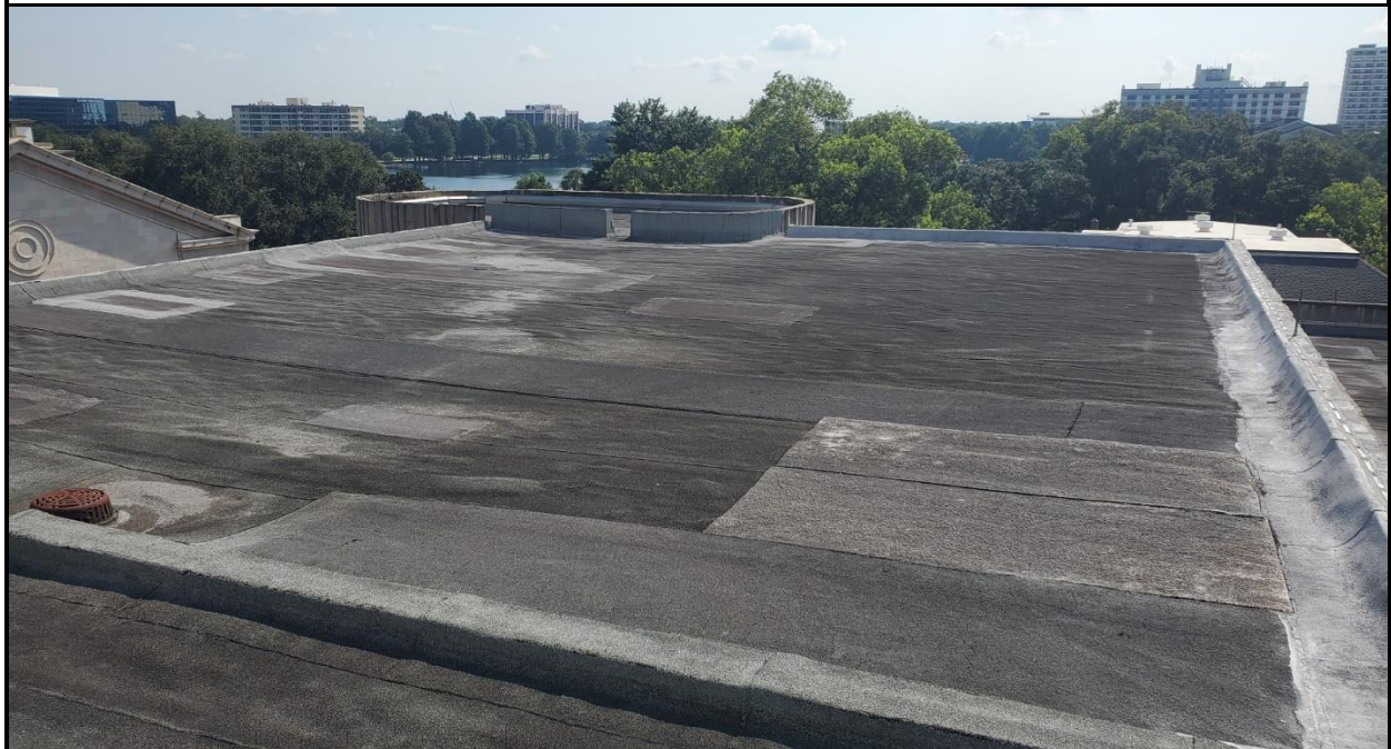
Photo 6: Overall view of roof area 1F
