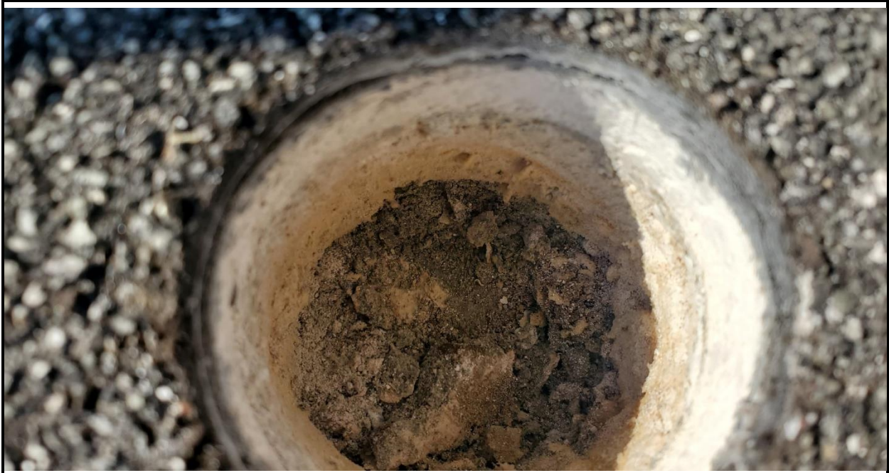
Photo 3: Roof core cavity of sample 1
