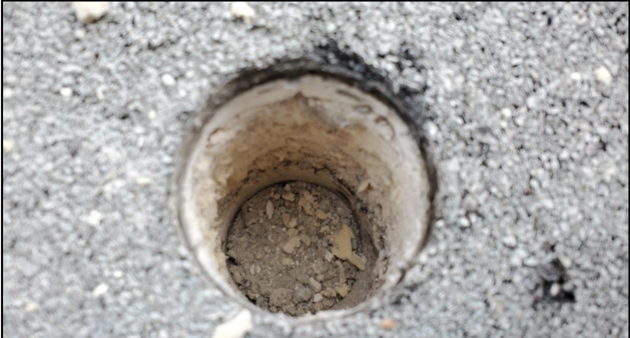
Photo 10: Roof core 3 collected from area 7E
