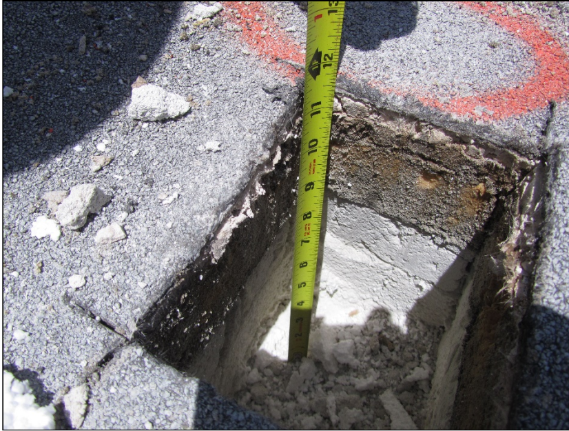
Photo 11: Roof Section 2 – Core Location A3 – Core thickness.
