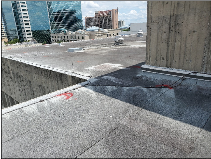
Photo 13: Overview of Roof Section 3.
