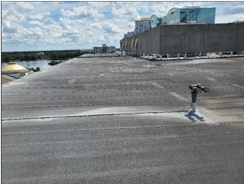
Photo 2: Overview of Roof Section 2.
