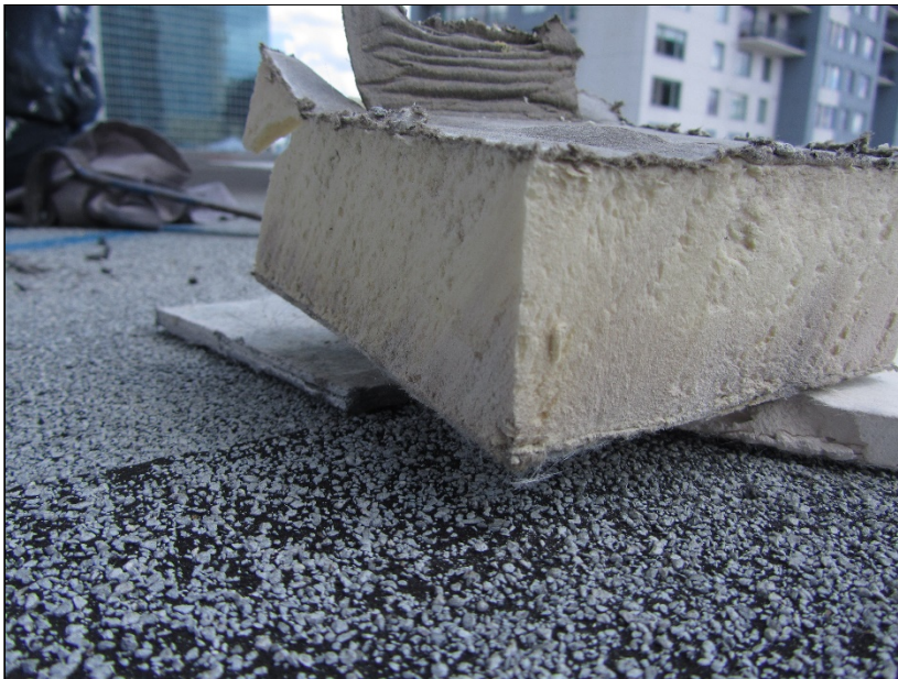
Photo 16: Roof Section 3 – Core Location L2 – polyiso insulation layer relatively dry.
