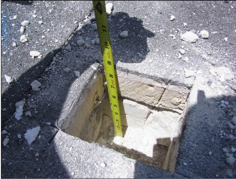
Photo 7: Roof Section 2 – Core Location C10 – Core thickness.
