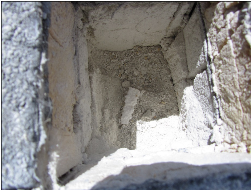
Photo 4: Roof Section 2 – Core Location N8 – roofing components relatively dry.
