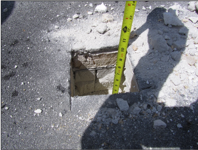
Photo 5: Roof Section 2 – Core Location N8 – Core thickness.
