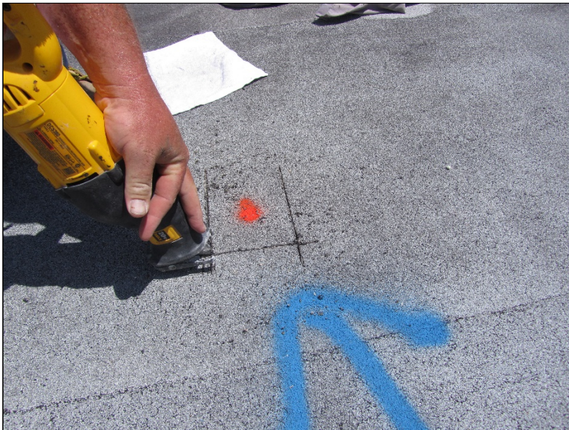
Photo 18: Roof Section 3 – Core Location B3 – coring in progress.
