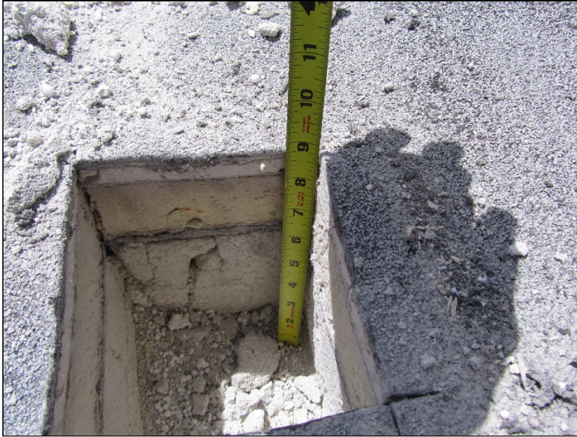
Photo 17: Roof Section 3 – Core Location L2 – core thickness.
