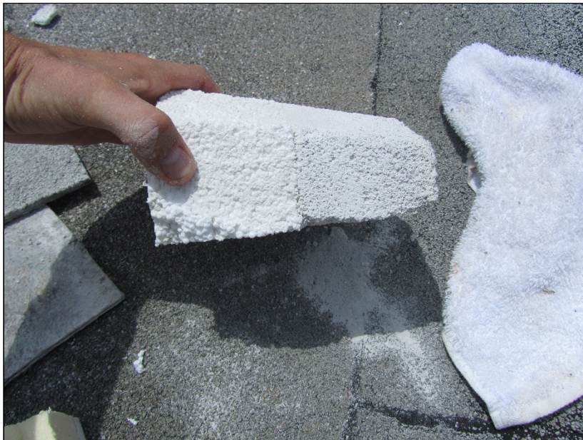
Photo 14: Roof Section 3 – Core Location F11 – relatively dry roofing components.
