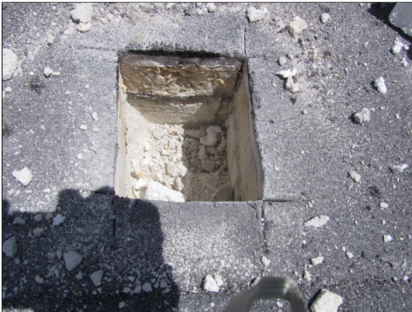
Photo 6: Roof Section 2 – Core Location C10 – relatively dry roofing components.
