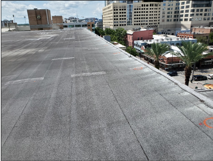
Photo 1: Overview of Roof Section 2.
