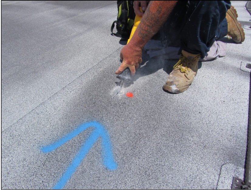
Photo 3: Roof Section 2 – Core Location N8 – Core in progress.
