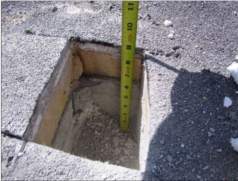
Photo 2: Roof Section 4 – Core Location J7.
