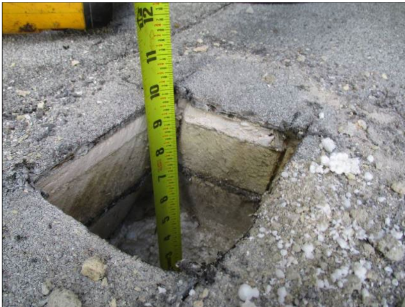
Photo 30: Roof Section 6A – Core Location B19.
