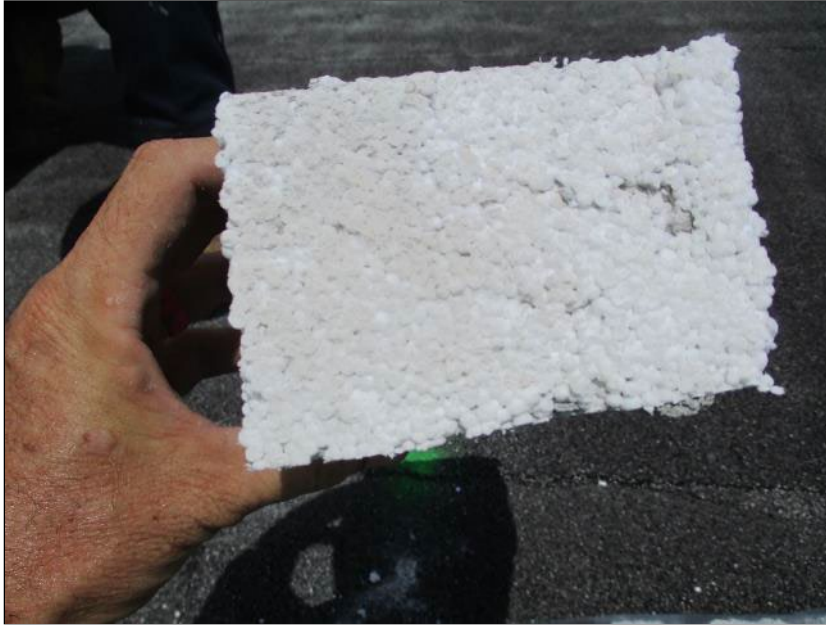
Photo 63: Roof Section 11 – Core Location B9.
