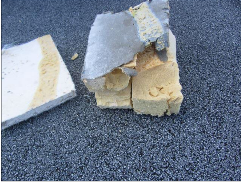
Photo 1: Roof Section 4 – Core Location J7.
