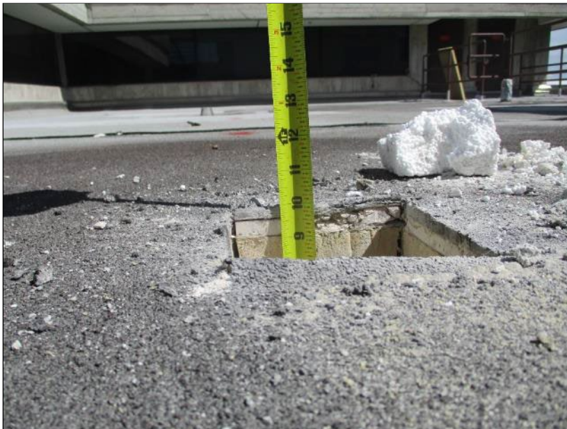
Photo 16: Roof Section 6 – Core Location AE10.
