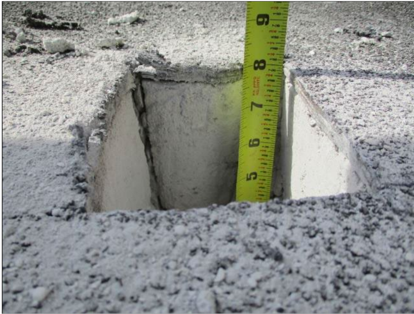
Photo 33: Roof Section 7/8 – Core Location G2.
