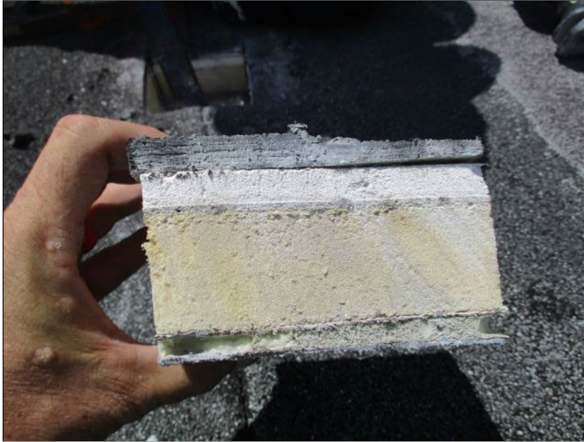
Photo 51: Roof Section 10 – Core Location Q5.
