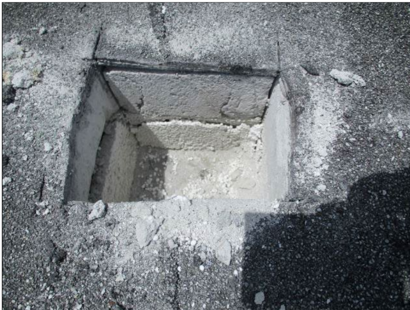
Photo 62: Roof Section 11 – Core Location B9.
