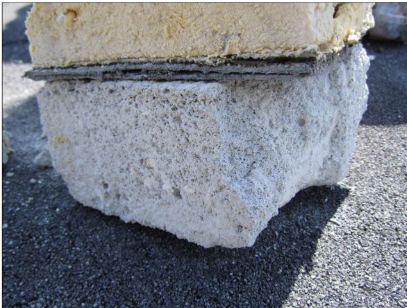
Photo 6: Roof Section 5 – Core Location E11.
