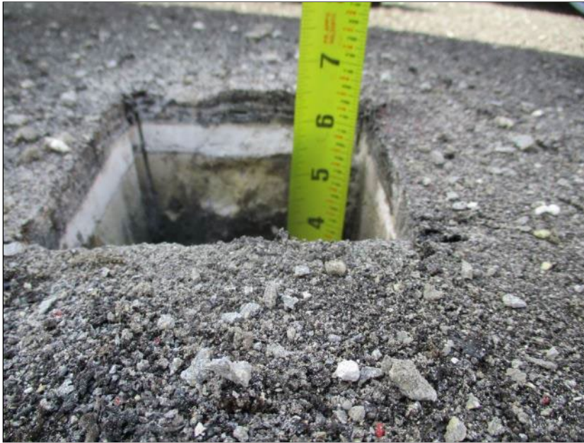
Photo 41: Roof Section 7/8 – Core Location F10.
