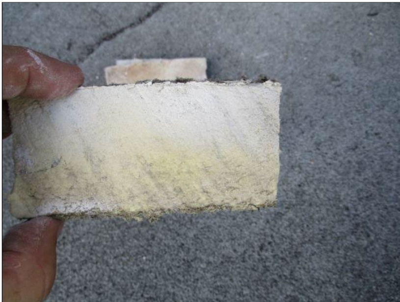
Photo 24: Roof Section 6A – Core Location B13.
