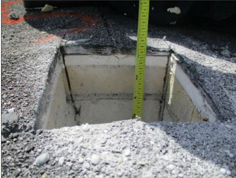
Photo 53: Roof Section 10 – Core Location Q5.
