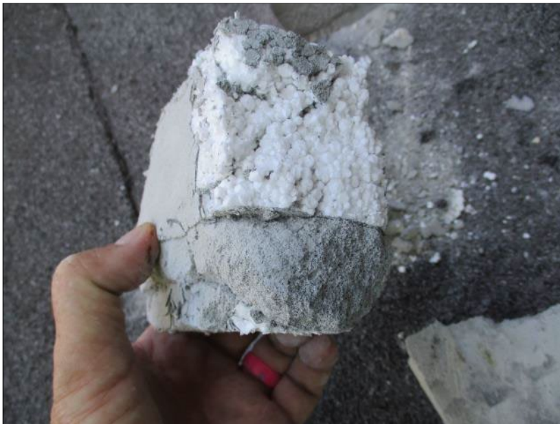
Photo 42: Roof Section 9 – Core Location B16.
