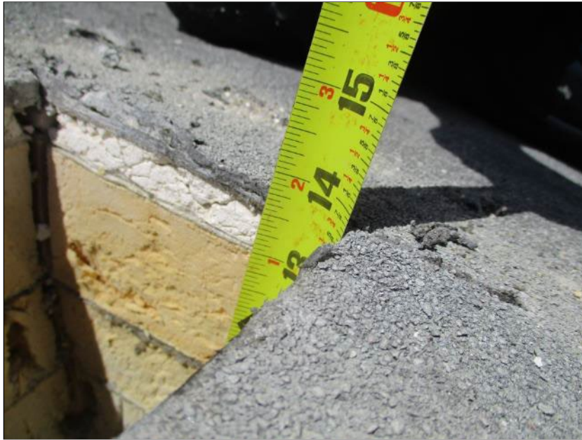
Photo 13: Roof Section 6 – Core Location N3.
