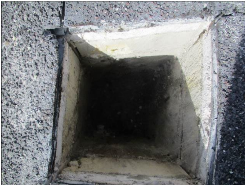
Photo 36: Roof Section 7/8 – Core Location H15.
