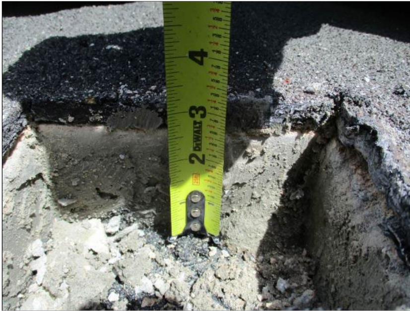
Photo 47: Roof Section 9 – Core Location C6.
