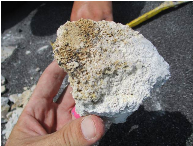
Photo 68: Roof Section 11 – Core Location E7.
