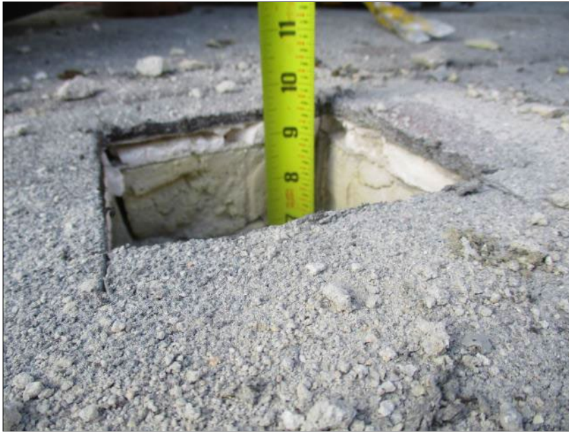
Photo 27: Roof Section 6A – Core Location B13.
