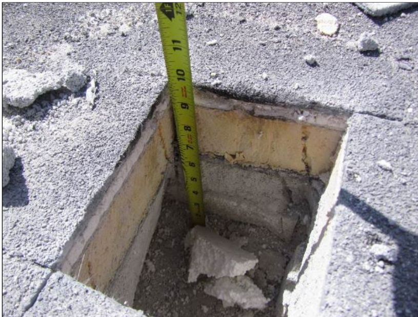
Photo 4: Roof Section 4 – Core Location B2.
