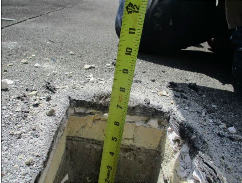
Photo 61: Roof Section 10 – Core Location E3.
