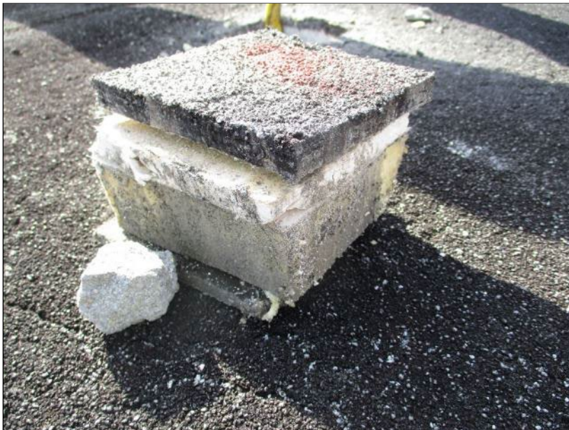
Photo 38: Roof Section 7/8 – Core Location F10.
