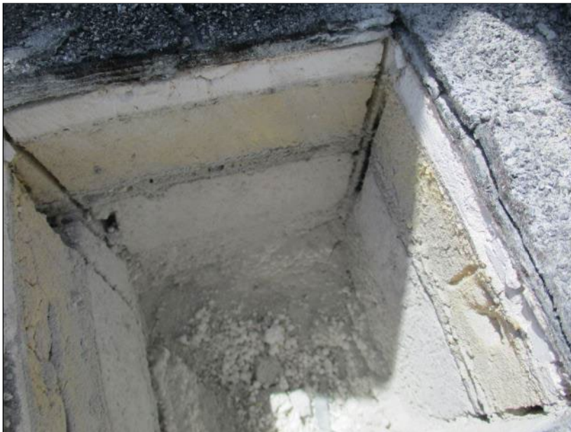
Photo 52: Roof Section 10 – Core Location Q5.
