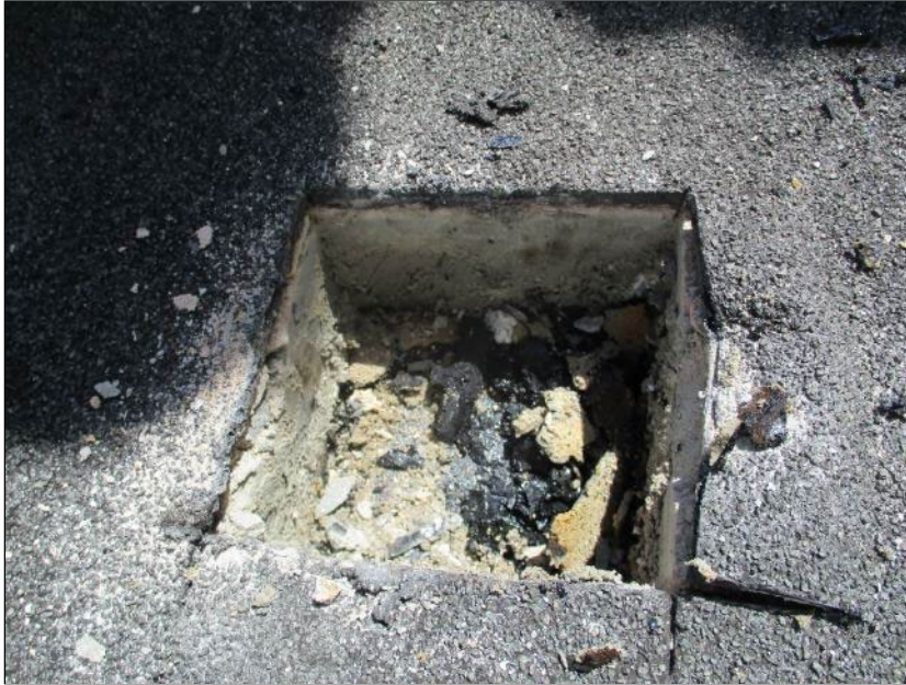
Photo 49: Roof Section 9 – Core Location B3.
