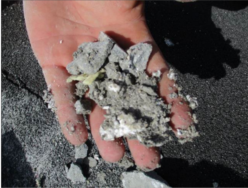
Photo 35: Roof Section 7/8 – Core Location H15.
