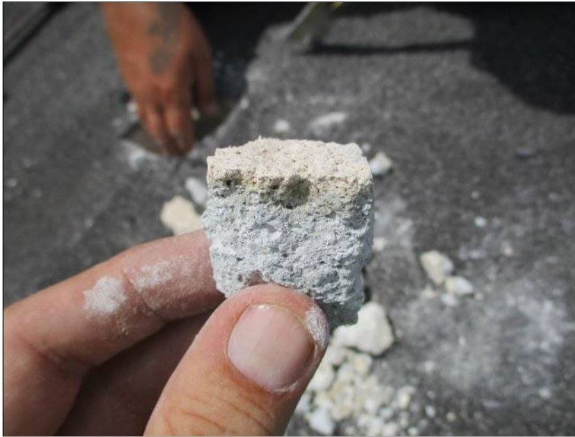
Photo 69: Roof Section 11 – Core Location E7.
