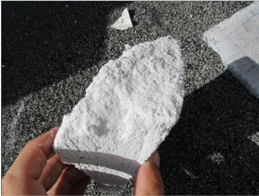
Photo 31: Roof Section 7/8 – Core Location G2.
