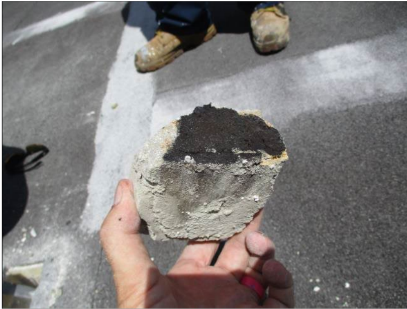
Photo 55: Roof Section 10 – Core Location G4.
