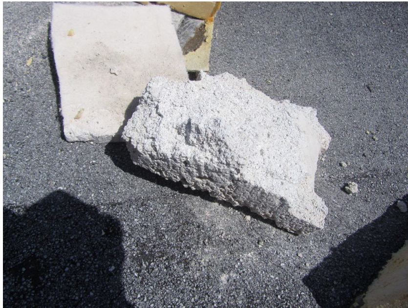
Photo 8: Roof Section 5 – Core Location E2.
