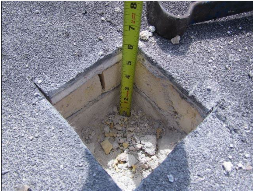
Photo 5: Roof Section 4 – Core Location G4.
