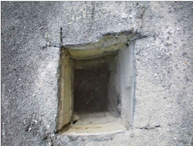
Photo 22: Roof Section 6A – Core Location A5.
