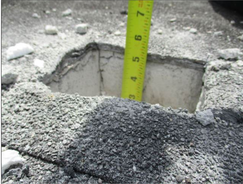
Photo 67: Roof Section 11 – Core Location J2.
