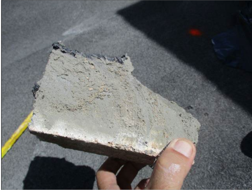
Photo 45: Roof Section 9 – Core Location C6.
