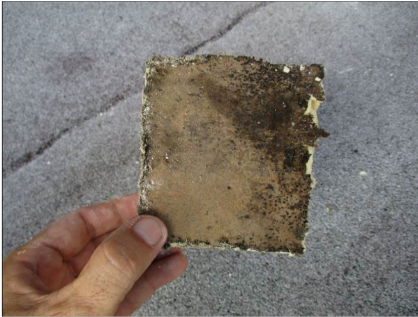
Photo 25: Roof Section 6A – Core Location B13.
