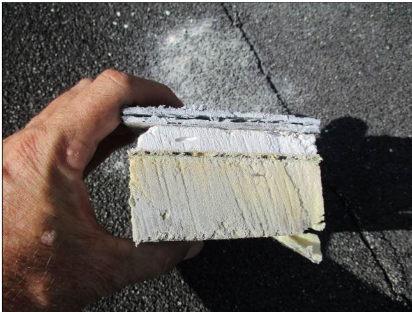
Photo 34: Roof Section 7/8 – Core Location H15.
