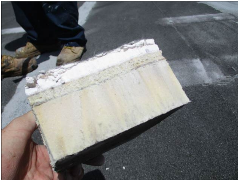
Photo 54: Roof Section 10 – Core Location G4.
