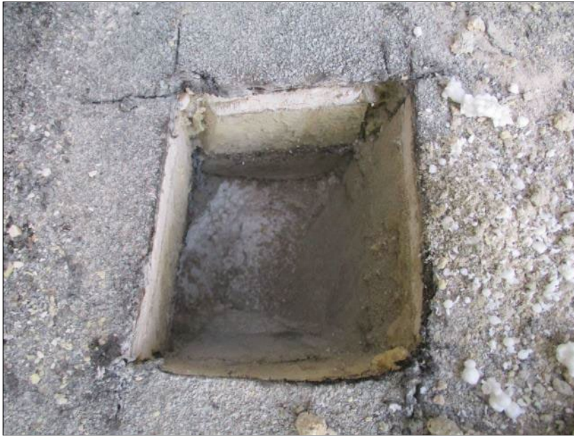
Photo 29: Roof Section 6A – Core Location B19.
