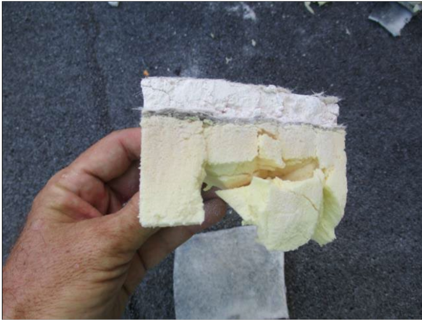
Photo 21: Roof Section 6A – Core Location A5.
