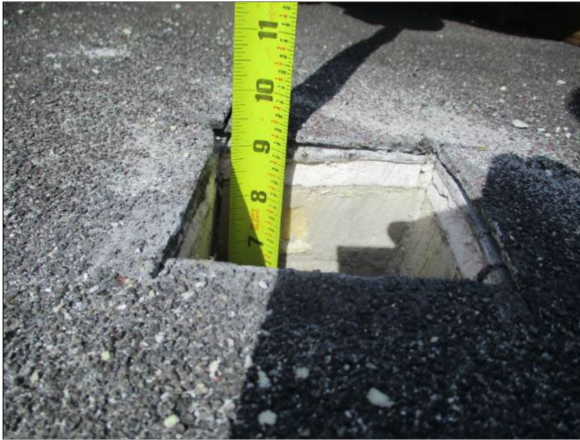
Photo 37: Roof Section 7/8 – Core Location H15.
