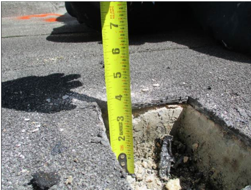
Photo 50: Roof Section 9 – Core Location B3.
