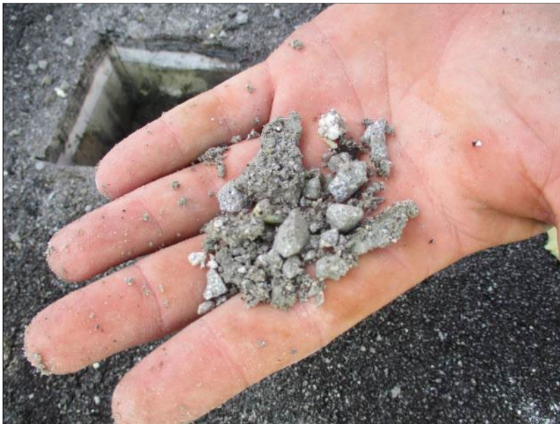
Photo 40: Roof Section 7/8 – Core Location F10.
