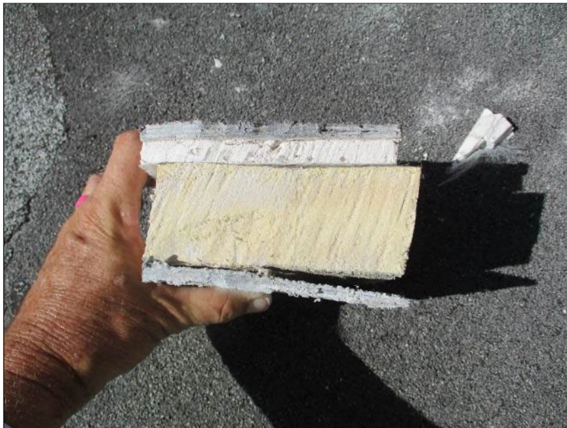
Photo 14: Roof Section 6 – Core Location AE10.
