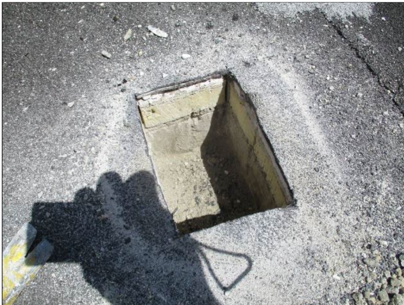
Photo 56: Roof Section 10 – Core Location G4.
