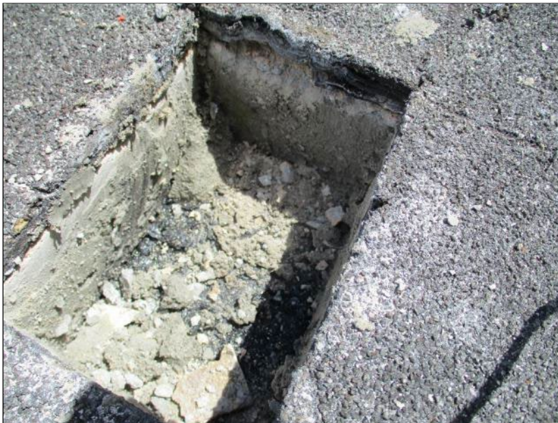
Photo 46: Roof Section 9 – Core Location C6.
