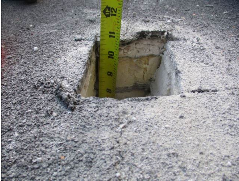
Photo 23: Roof Section 6A – Core Location A5.
