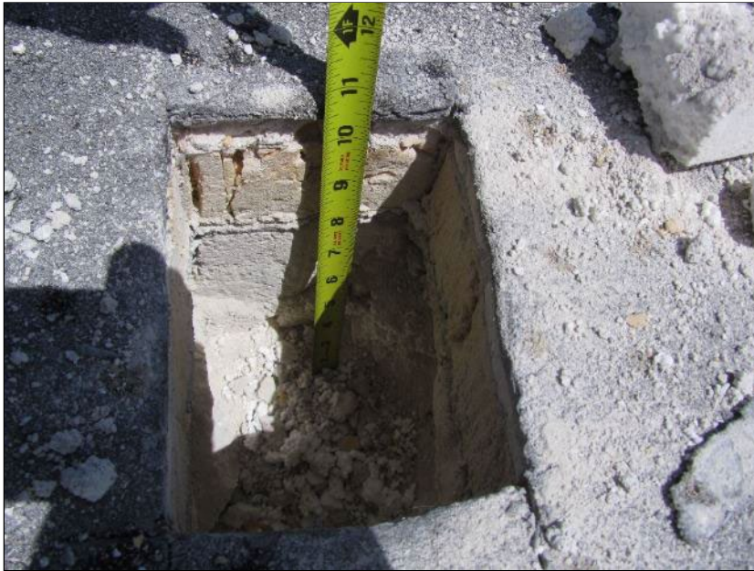
Photo 9: Roof Section 5 – Core Location E2.
