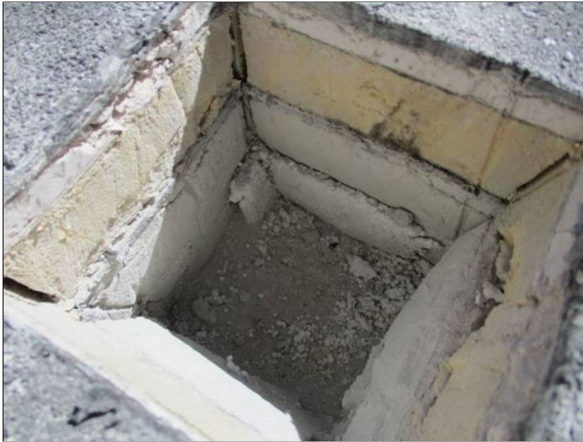
Photo 15: Roof Section 6 – Core Location AE10.
