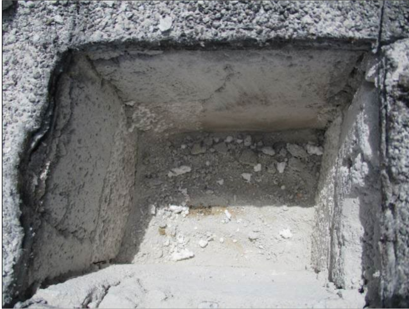
Photo 65: Roof Section 11 – Core Location J2.
