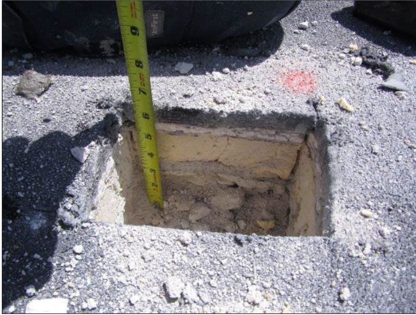
Photo 11: Roof Section 5 – Core Location D6.
