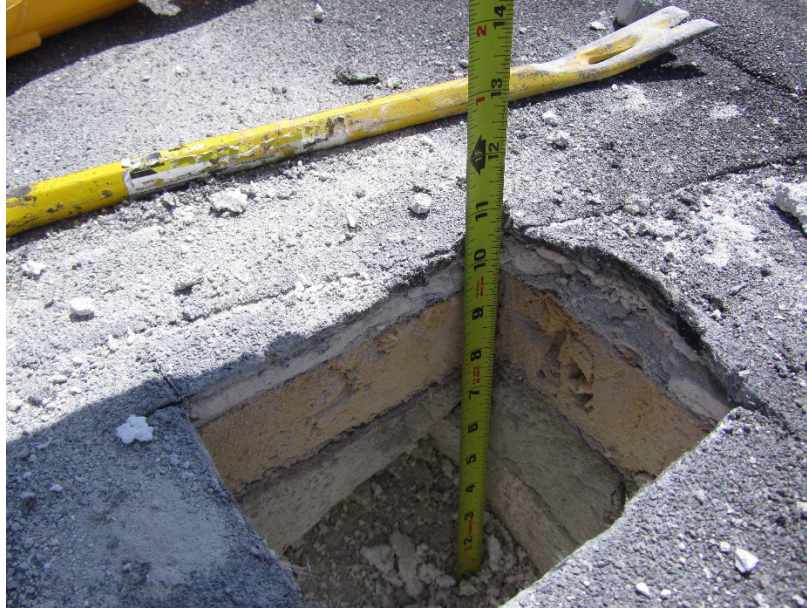
Photo 7: Roof Section 5 – Core Location E11.
