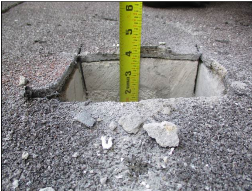
Photo 44: Roof Section 9 – Core Location B16.
