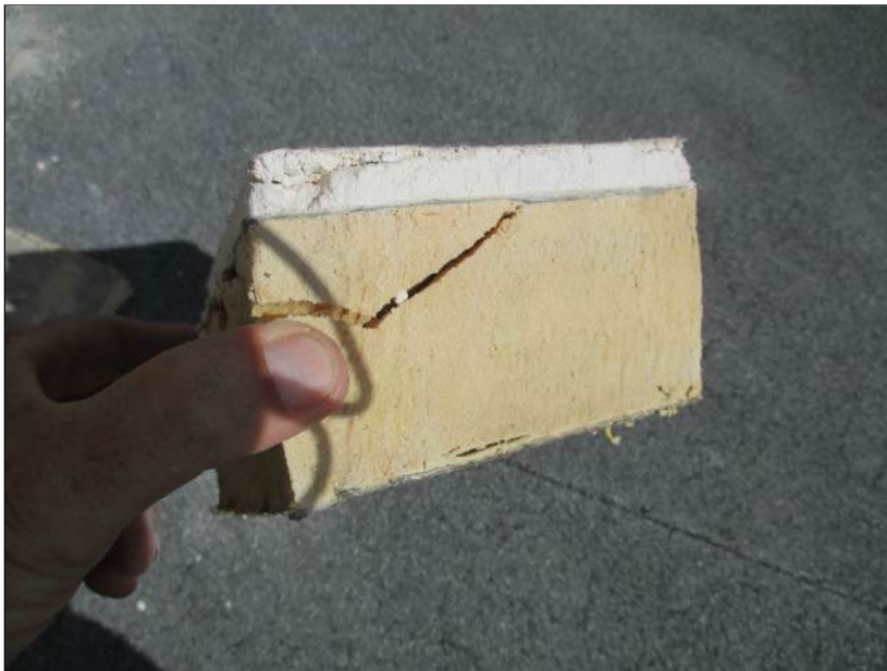
Photo 12: Roof Section 6 – Core Location N3.
