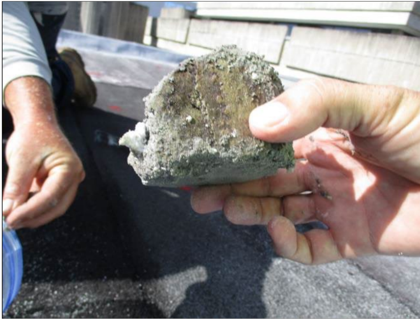
Photo 39: Roof Section 7/8 – Core Location F10.
