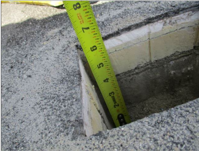
Photo 57: Roof Section 10 – Core Location G4.
