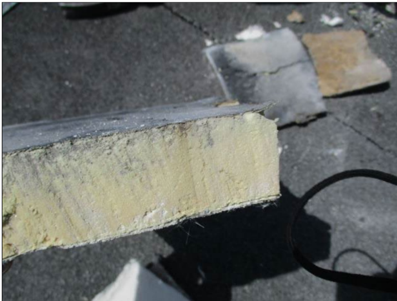
Photo 58: Roof Section 10 – Core Location E3.
