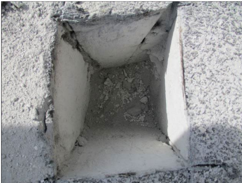
Photo 32: Roof Section 7/8 – Core Location G2.
