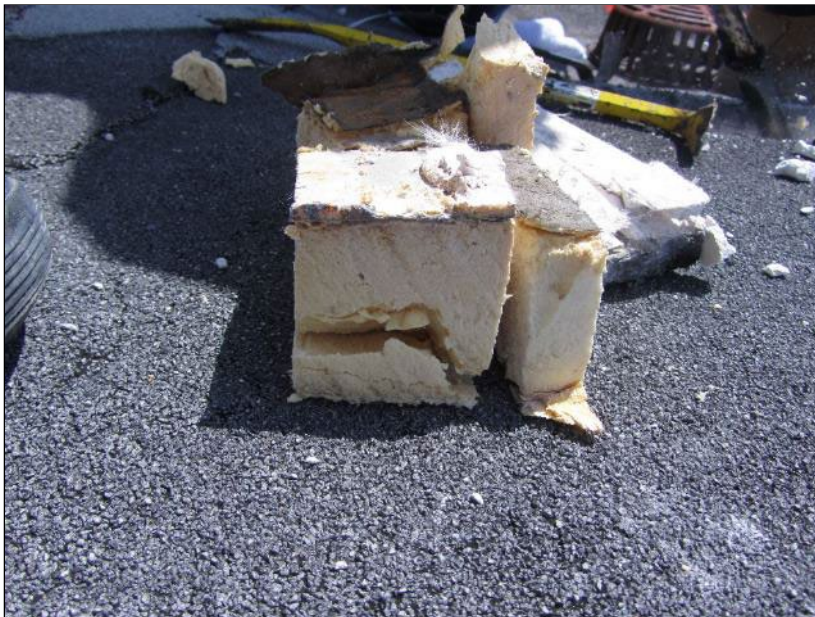
Photo 10: Roof Section 5 – Core Location D6.
