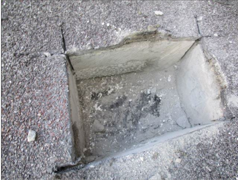
Photo 43: Roof Section 9 – Core Location B16.
