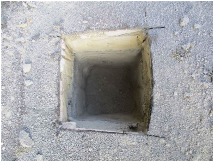
Photo 26: Roof Section 6A – Core Location B13.
