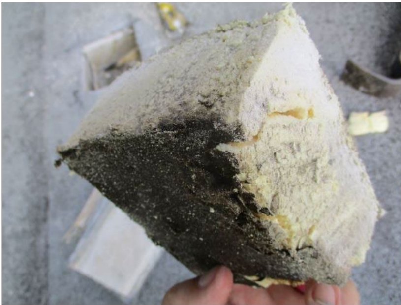
Photo 28: Roof Section 6A – Core Location B19.
