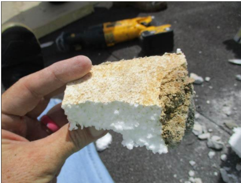
Photo 66: Roof Section 11 – Core Location J2.
