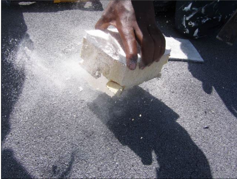
Photo 3: Roof Section 4 – Core Location B2.
