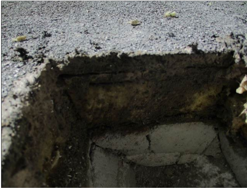
Photo 19: Roof Section 6 – Core Location C10.
