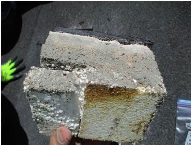
Photo 48: Roof Section 9 – Core Location B3.
