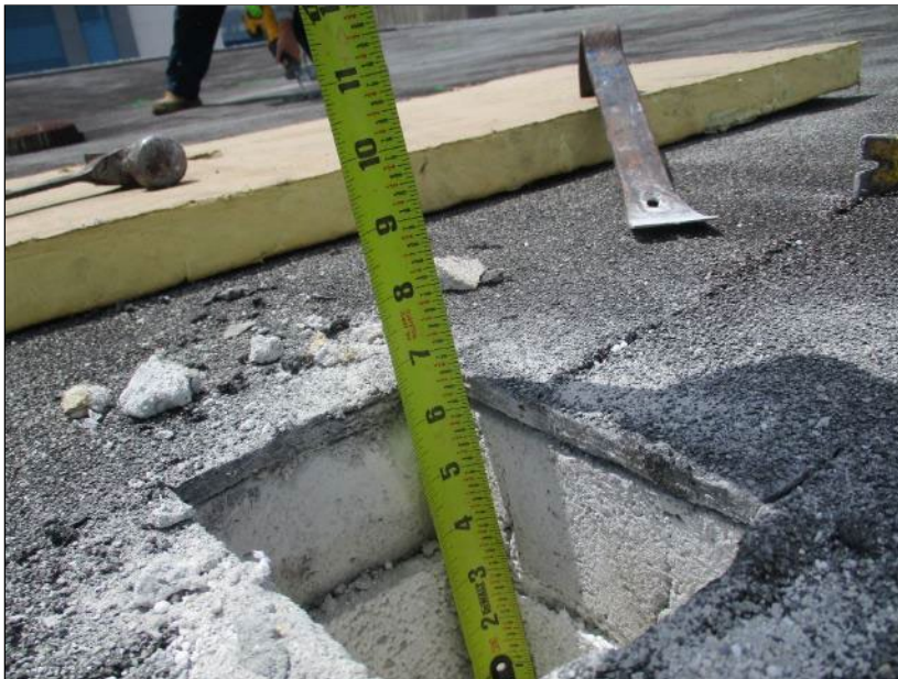
Photo 64: Roof Section 11 – Core Location B9.
