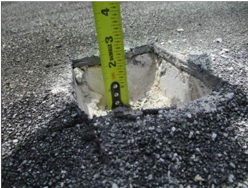
Photo 70: Roof Section 11 – Core Location E7.
