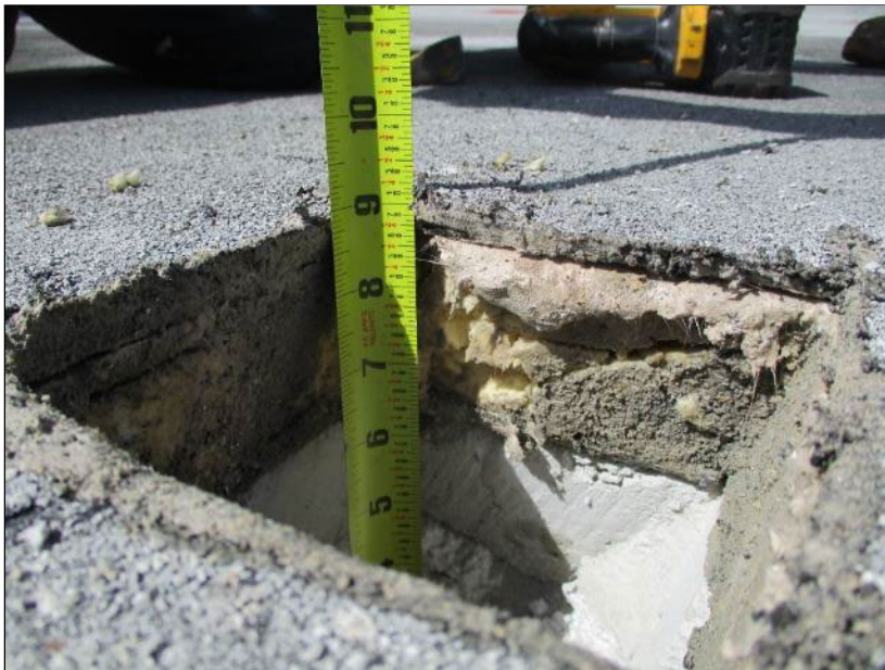
Photo 20: Roof Section 6 – Core Location C10.
